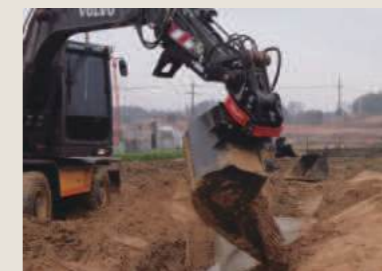
Backfilling
